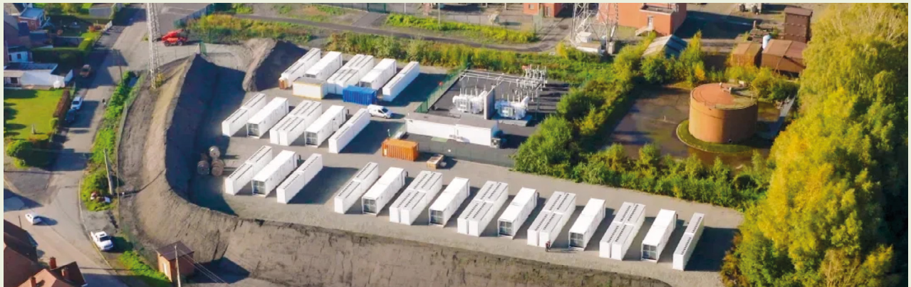
Figure 18: Drone Shot of Deux Acren During Building Phase
